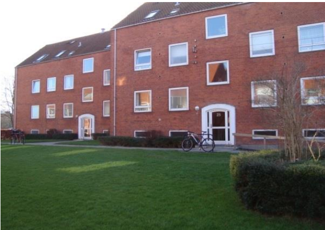
Original Danish Pilot – Riffelhavevej
