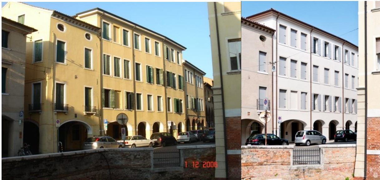
General view of the building before and after the intervention
