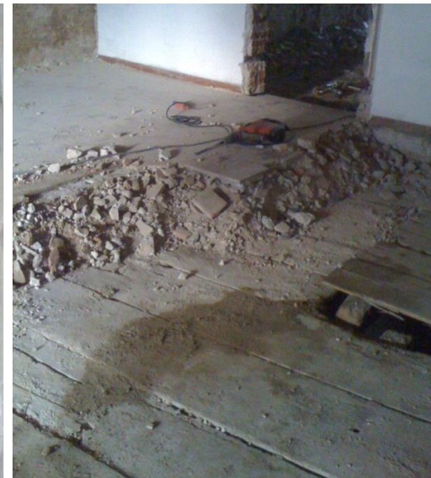
Demolished partition walls left and used as a substrate
