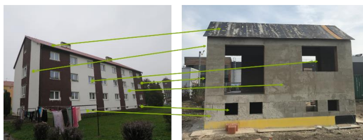
Figure 1. Original pilot building in the left and the mock-up house built up for the RLLL setup
