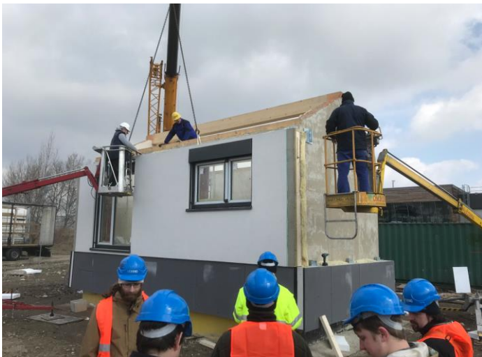
Figure 7. Integrated wall module placement (noon)
