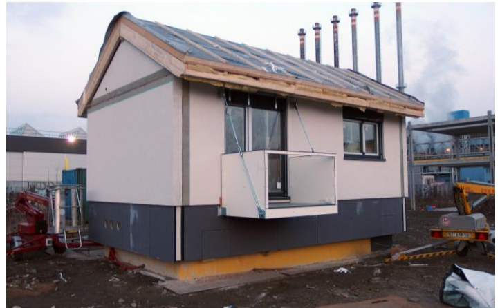
Figure 10. End of installation (8 p.m.)
