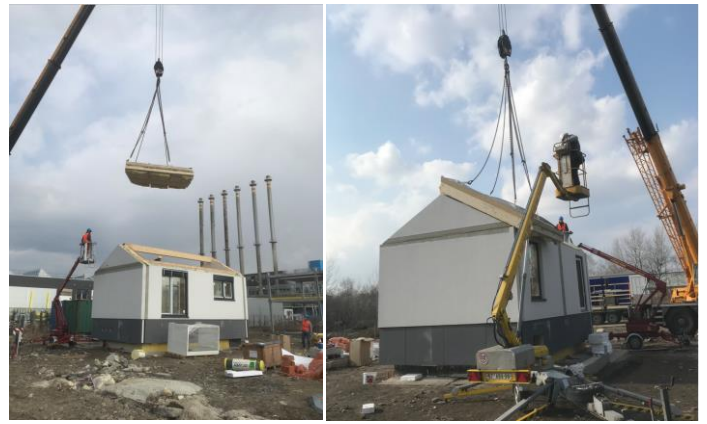
Figure 8. Placement of roof modules (4 p.m.)
