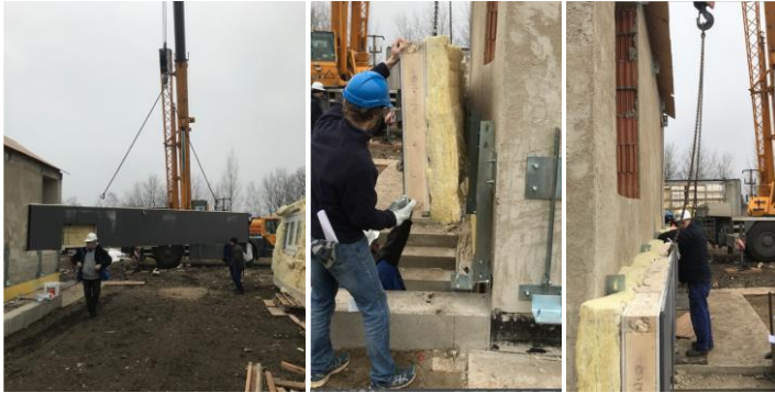
Figure 5. Installation of modules (8 a.m.)
