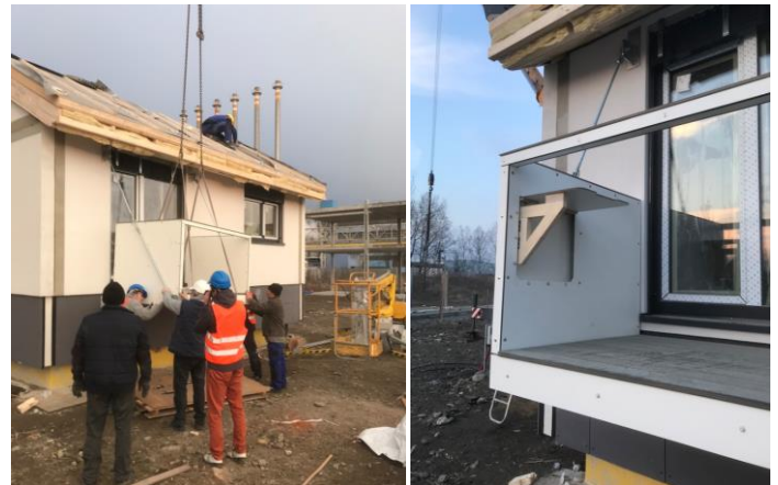
Figure 9. Mountage of additional balcony (7 p.m.)
