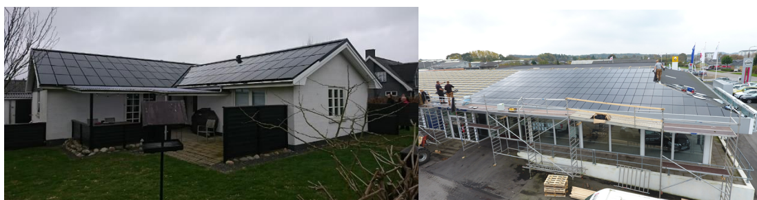
Two test sites for the INNOGIE integrated PV roofs
