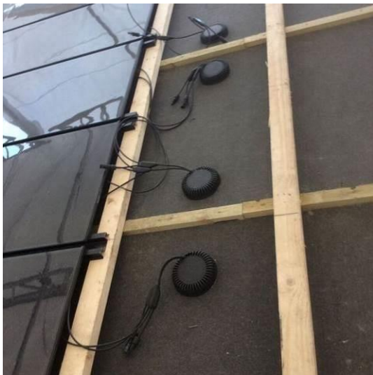
Figure 3.14: The cable is led through the underlying roof to the inside loft before the last PV-modules are mounted.
