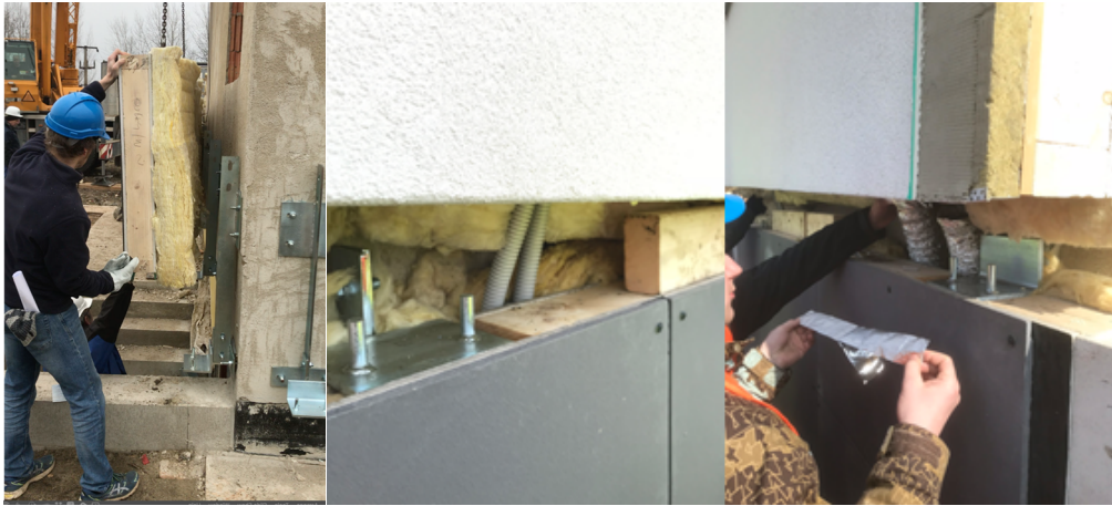
Figure 2.19 Installation of modules (8 a.m.-11 a.m.) and HVAC connections between the modules
