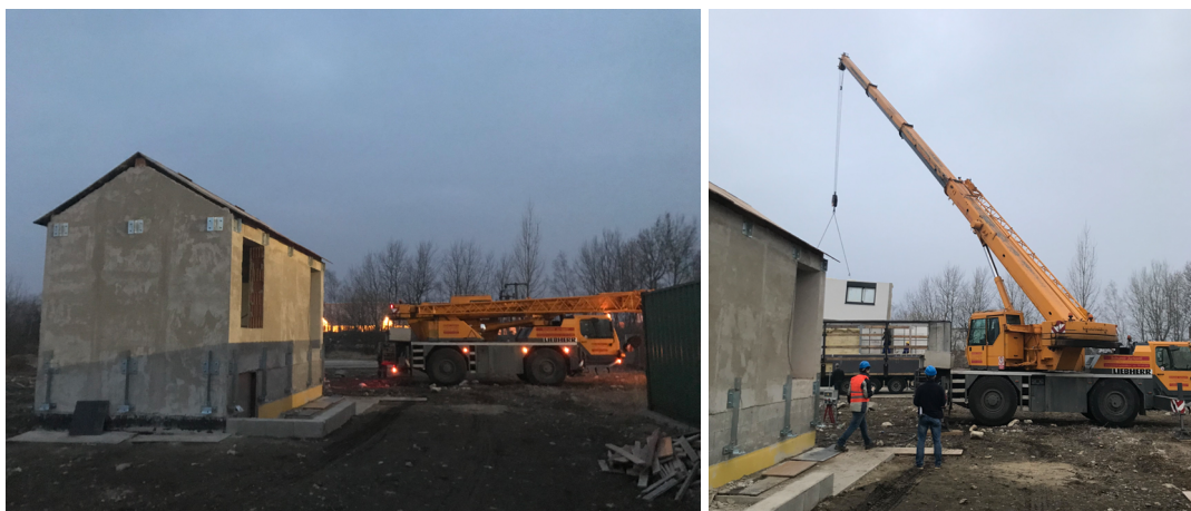
Figure 2.18 Installation: 6 a.m.: Prepared anchors on the simulated original building's façade. Unloading the first modules.
