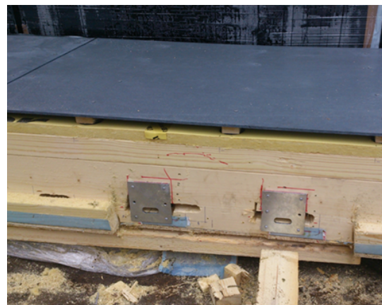
Figure 4.6 Steel brackets, 3D adjustable, for wall modular elements: designed solution (above left); brackets installed onto the wall (above right and below left); brackets support adjustment on the element before mounting at the pilot building site (below right)
