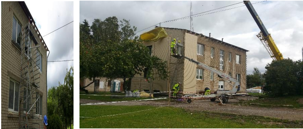
Figure 5.12 Use of scaffolding and crane lifting for the retrofitting work process
