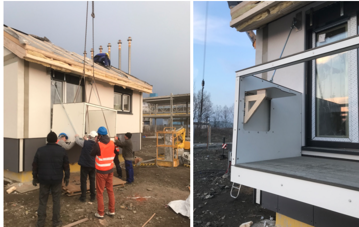
Figure 2.22 Montage of additional balcony (7 p.m.)
