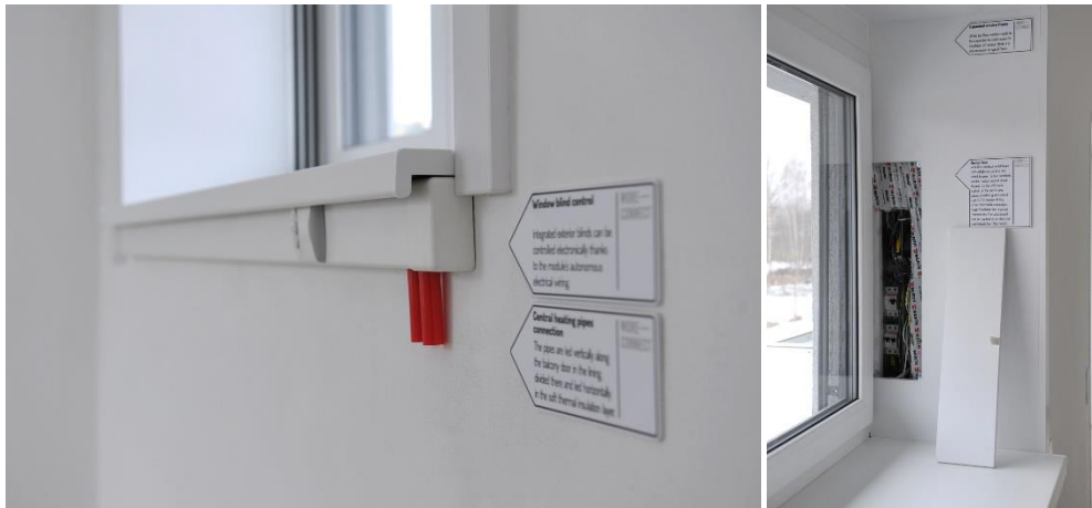
Figure 2.25 Information arrows for the demonstration purposes: hydronic heating preparation and window blinds' control element (left); window siding with electrical switchbox (right)
