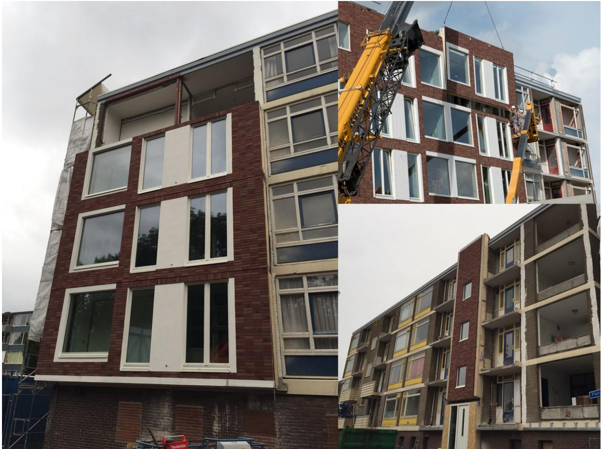
Figure 6.9 Installation of pre-fabricated wall elements at the Presikhaaf project.
