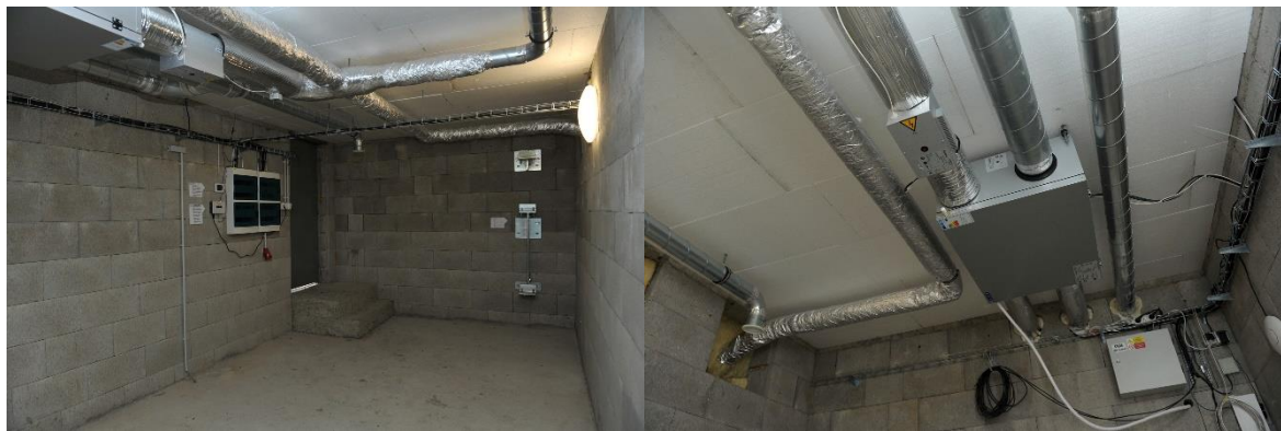
Figure 2.26 Engine room in the underground floor with ventilation unit.
