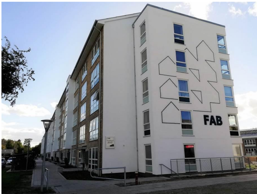
Figure 3.6 The insulated gable wall (25 cm rockwool) made with concrete finishing and robot-made decoration.
