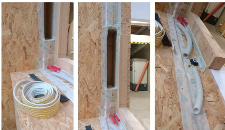
Figure 2.10 Development of air tight detail of electrical box installation.
