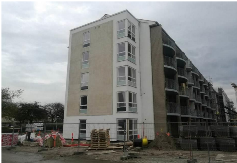
Figure 3.4 The insulated gable wall (25 cm Rockwool) ready for the concrete finishing and robot decoration painting.
