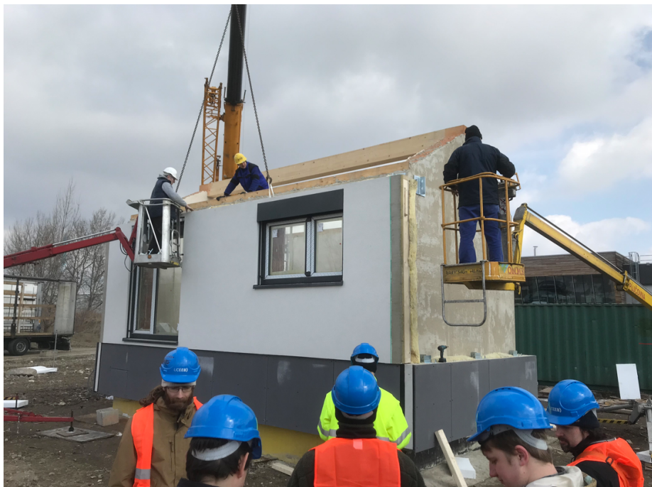
Figure 2.20 Integrated wall module placement (noon)
