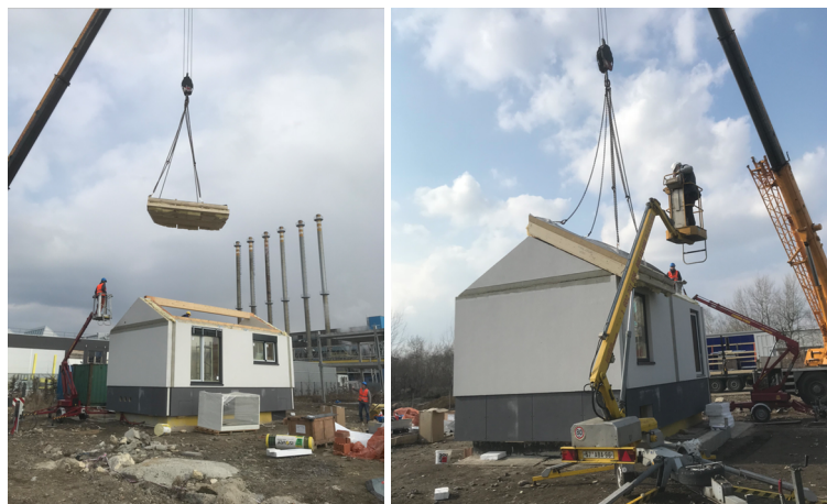
Figure 2.21 Placement of roof modules (4 p.m.)
