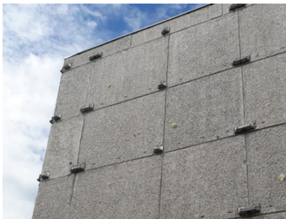
Figure 4.6 Steel brackets, 3D adjustable, for wall modular elements: designed solution (above left); brackets installed onto the wall (above right and below left); brackets support adjustment on the element before mounting at the pilot building site (below right)
