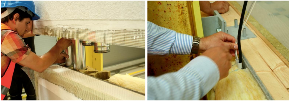
Figure 2.16 Connecting the HVAC tubes with inserted elements (left) and installation of cables (right). This might be quite dangerous manoeuvre in windy conditions on site, perhaps some kind of provisional wedges or other kind of distance keeper shall be inserted between the panels before the workers work with their hands between the modules. This way turned out to be impractical and delaying the installation works. Would be better to have the cables in tight conduits so that they are stiff and slide easily into the slightly wider conduit in the lower panel.
