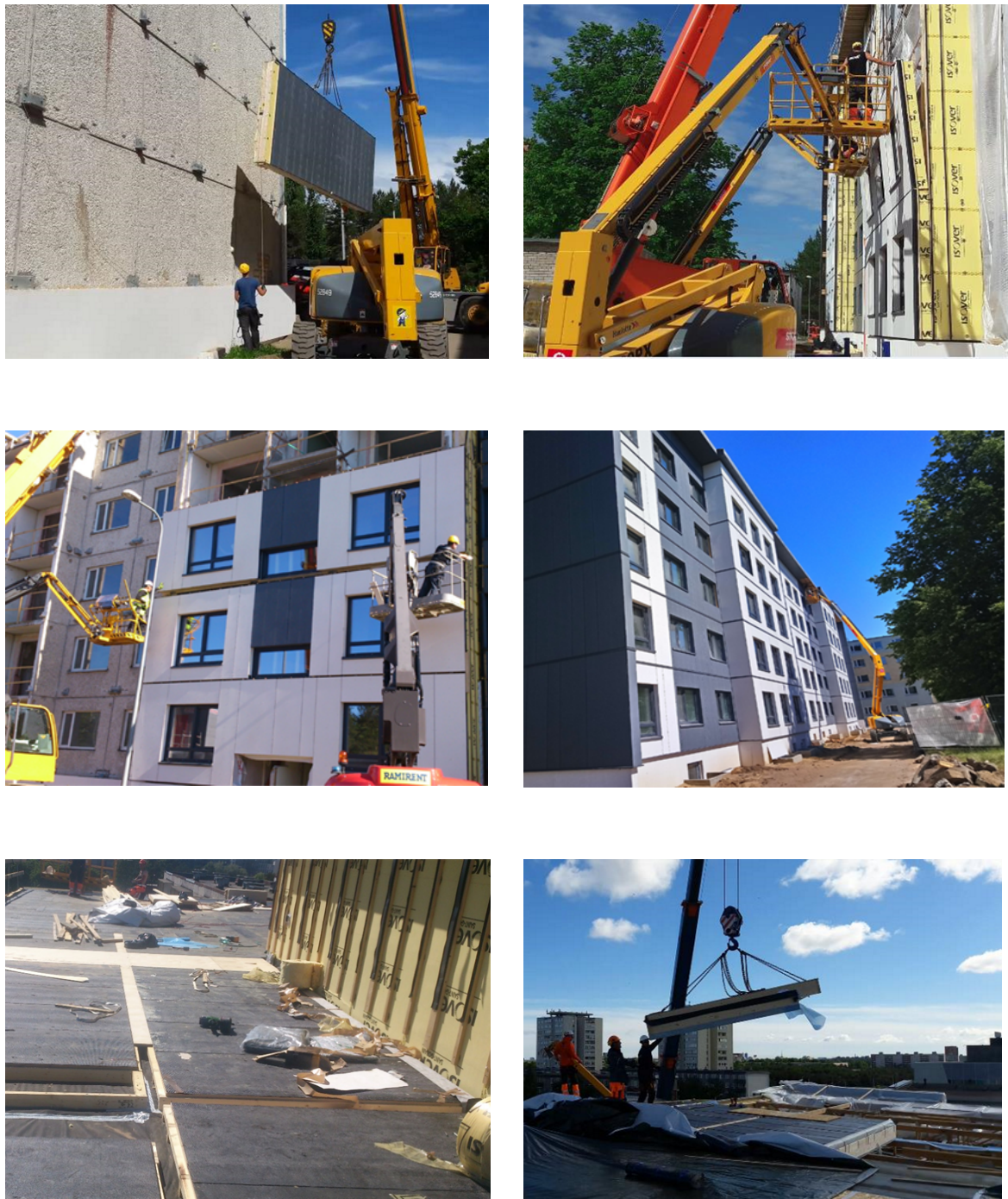
Figure 4.7 Mounting of wall (above and centre) and roof (below) modular elements at the building site (May-June 2017)
