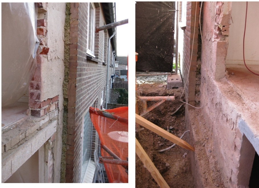
Figure 7.1 Connection between existing structures and new elements
